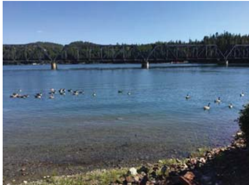
Looking upstream towards River left anchors from collection point.
