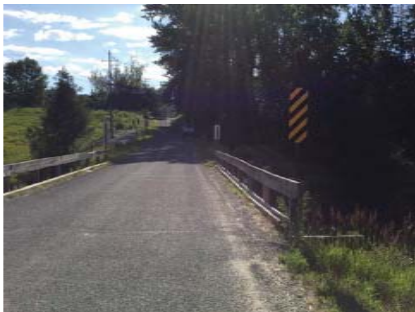
East view of bridge and small parking area.
