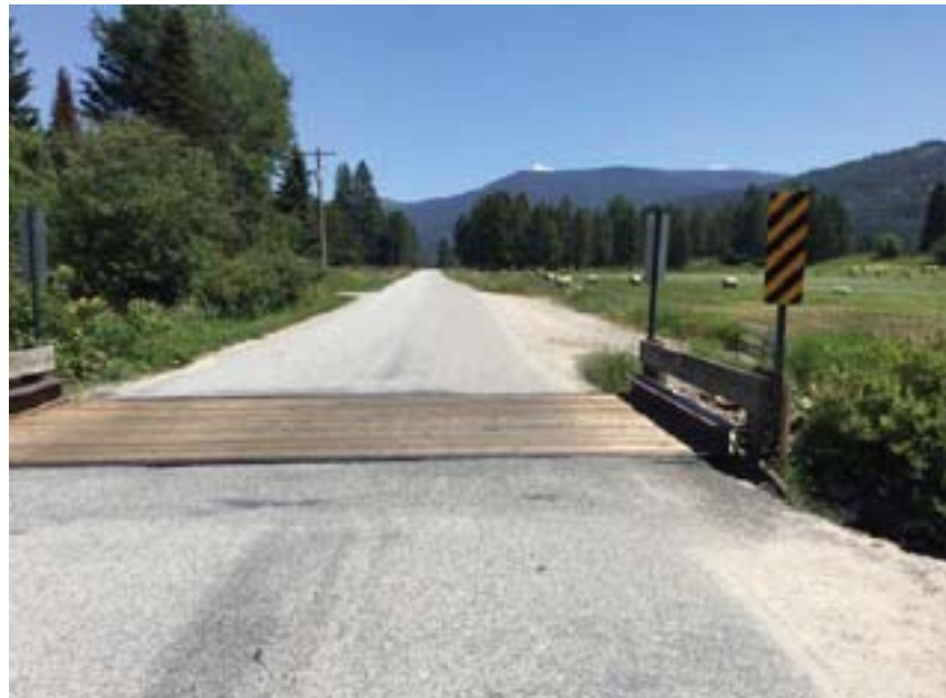
Looking east across bridge at parking area.
