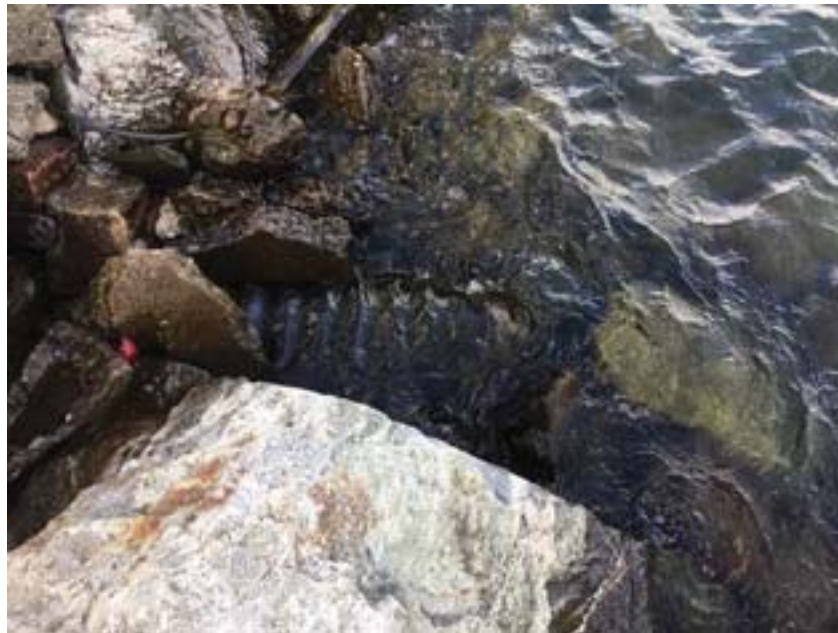
View of culvert.
