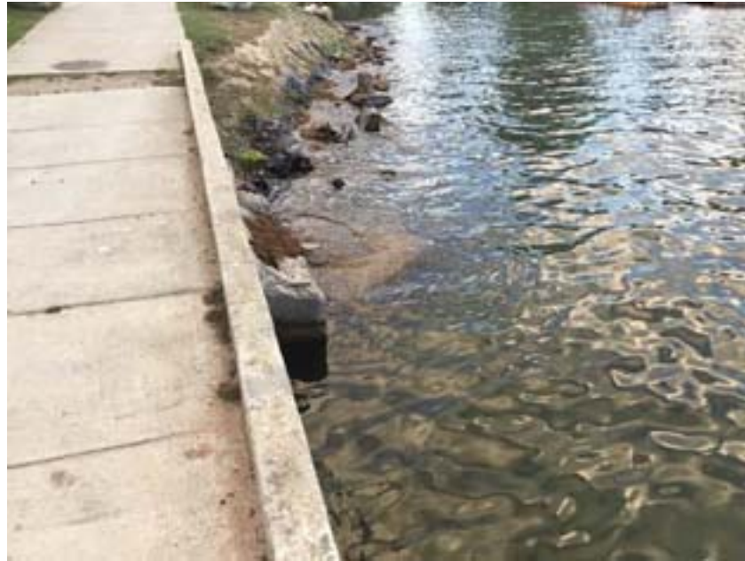
Image of concrete submerged culvert.
