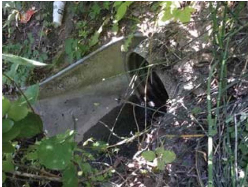
Concrete culvert on shoreline of river, but still difficult to access from water. Closest to Visitor Center.
