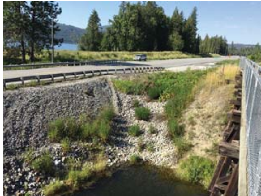
Small pullout on west side of bridge.
