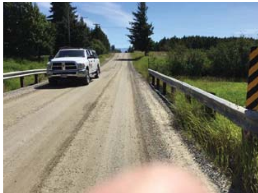
Looking east across bridge.
