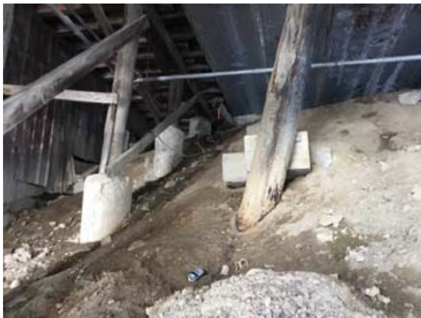
View of the southern culvert under bridge/restaurant.
