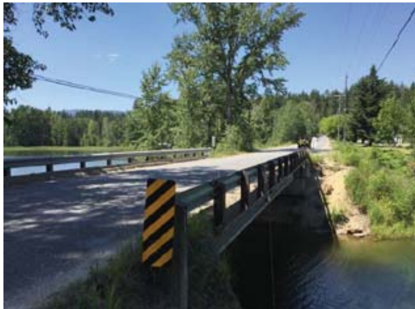
Bridge and narrow shoulders for parking.
