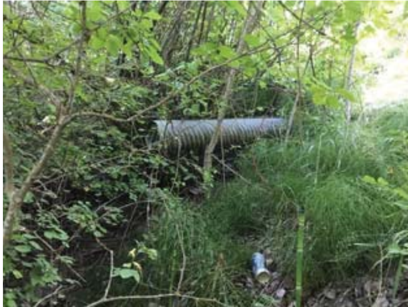
Metal pipe culvert 10+ ft from shore up embankment. Pipe diameter 8 inches.
