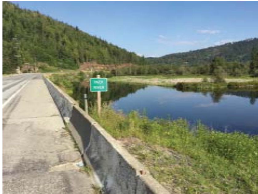
Pack River bridge from SR200 west bound.
