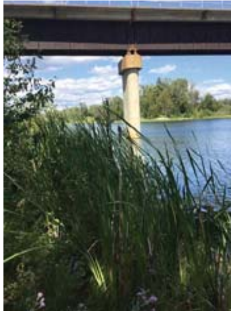
Picture taken from culvert facing upstream, rail link bridge in background for orientation.
