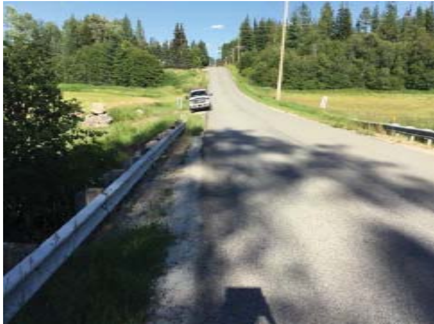
Sand creek looking north.
