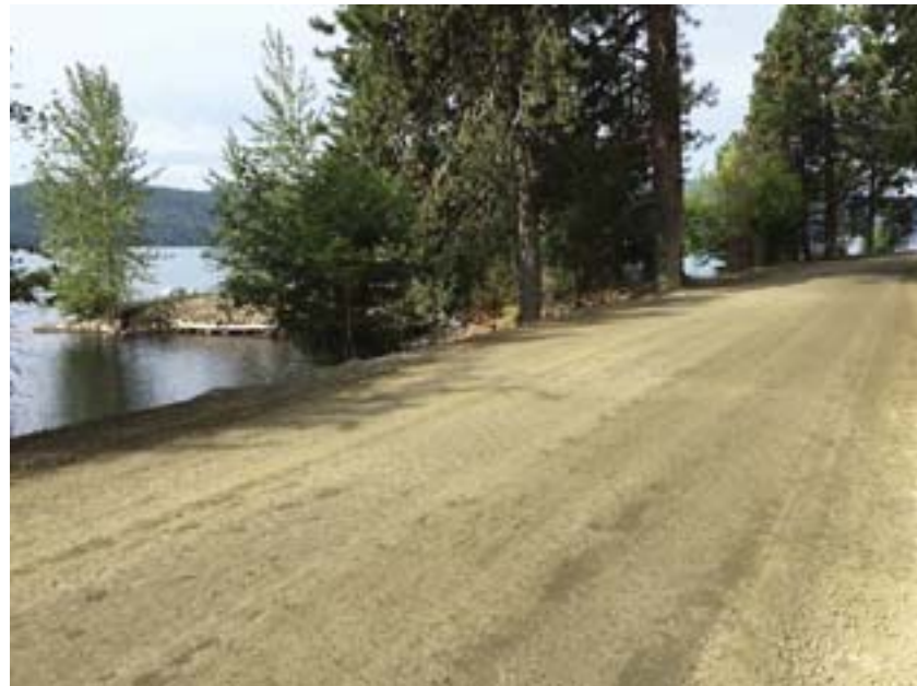
Staging area looking west.
