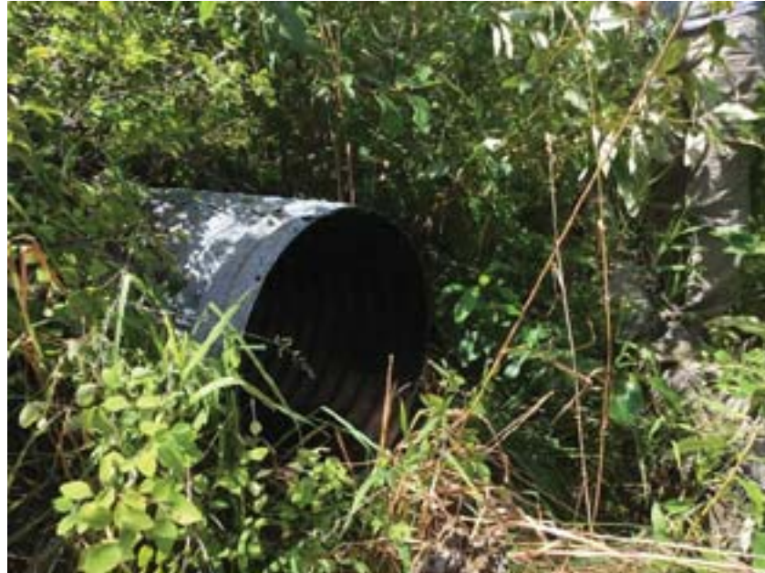
14 inch culvert South of railroad trestle.
