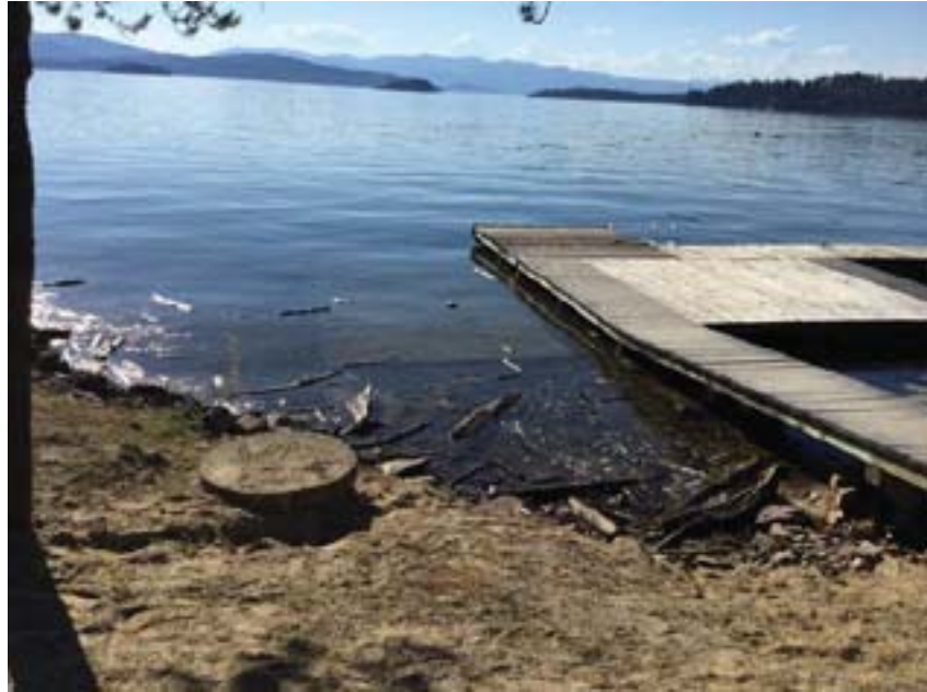
Surface water intake.
