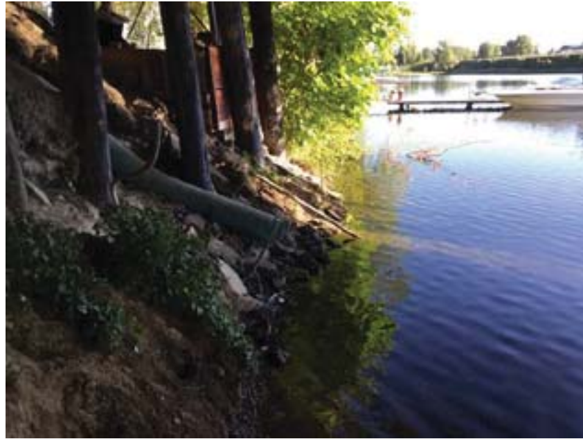
Image of concrete submerged culvert.
