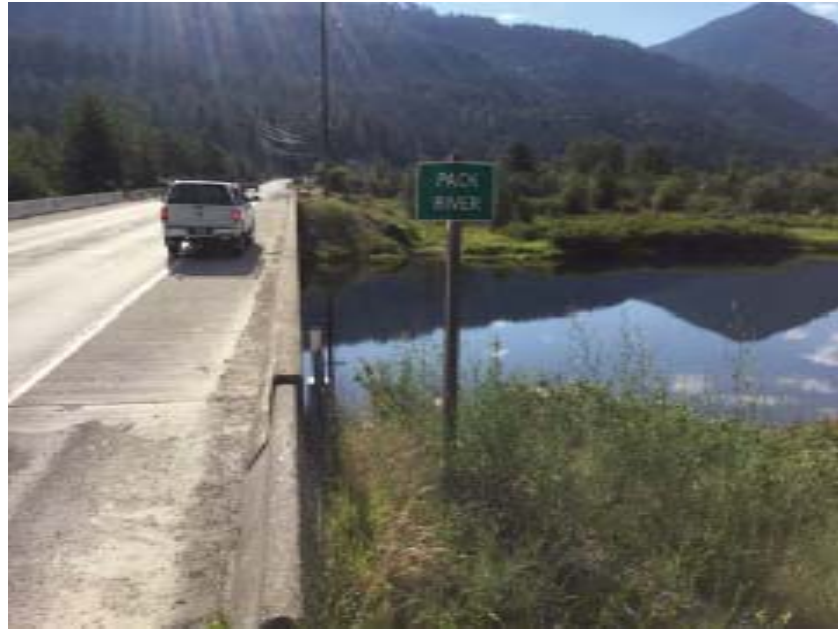
Pack River bridge from SR200 east bound.
