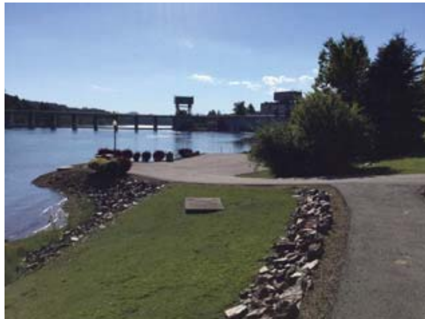
View of lower parking area with good vac truck access.
