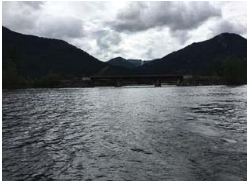
Looking South, towards Johnson Creek road bridge over Clark Fork South braid.
