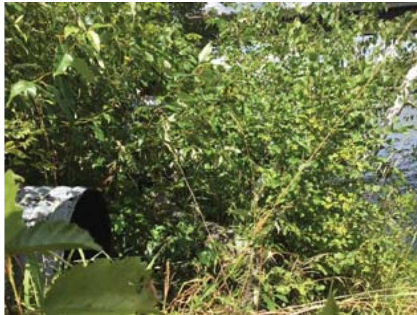
Picture of culvert facing downriver.
