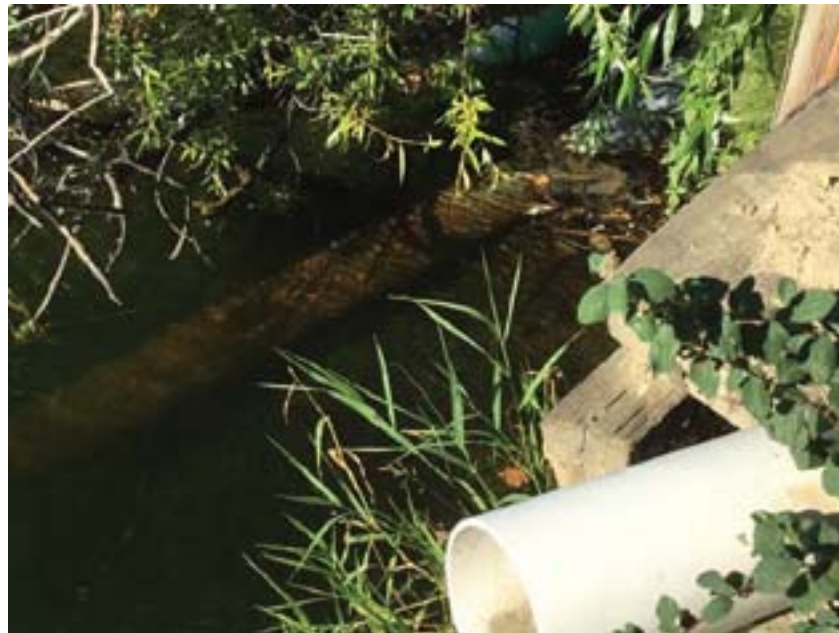
View from north of culverts facing south.
