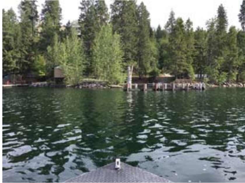
Looking north at water intake and anchor locations.
