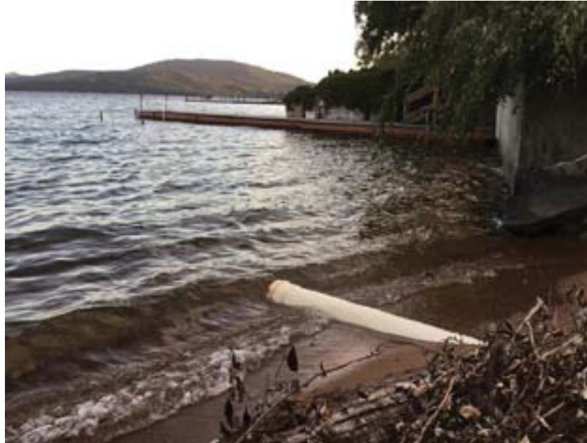
View looking south from north of culvert.
