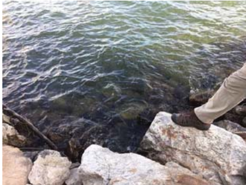
View of culvert. Currently underwater, but fluctuates with lake level from dam use.
