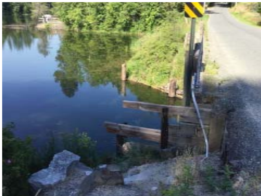
Downstream view of slough from the east side of bridge.
