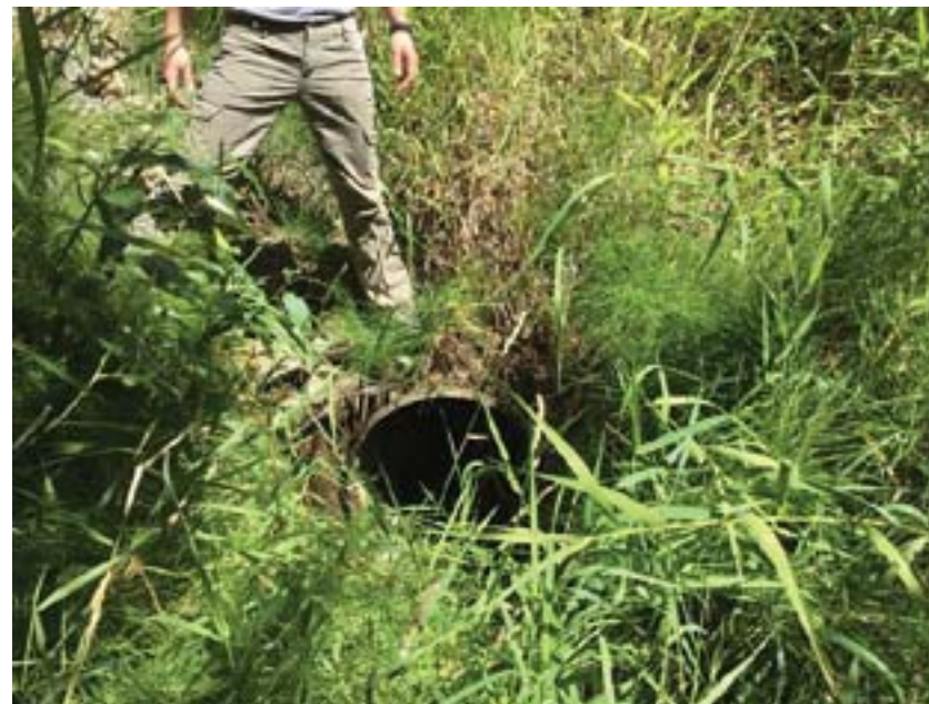
Facing east directly in front of culvert.
